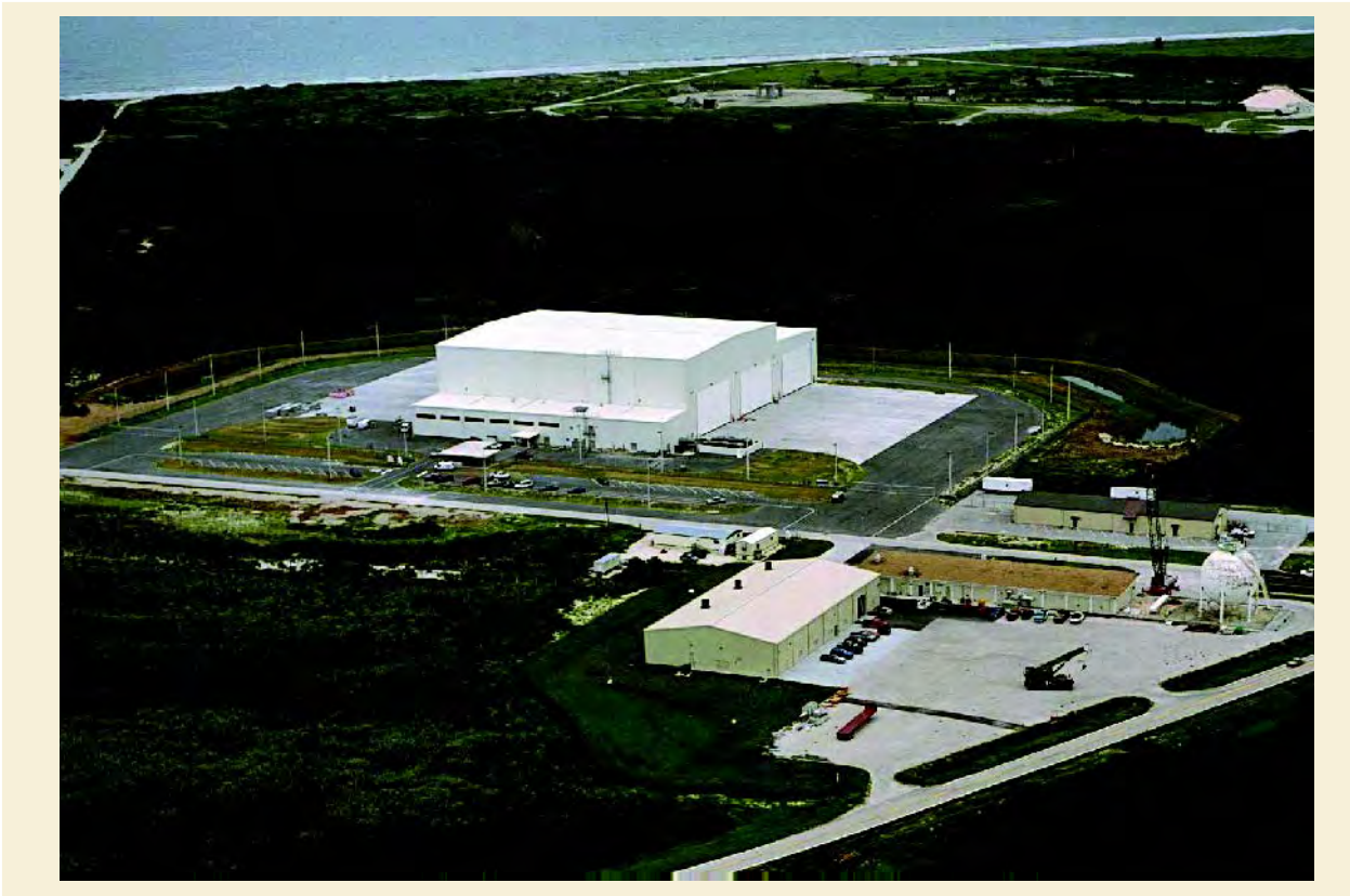
Figure 7-16. Space Launch Complex 37, Horizontal Integration Facility—Aerial View
